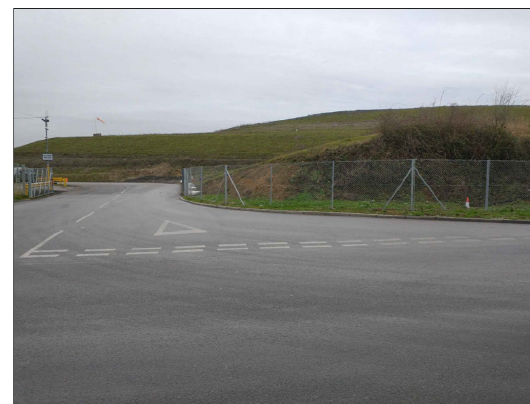
Looking west towards the left hand turn lane of the improved access
